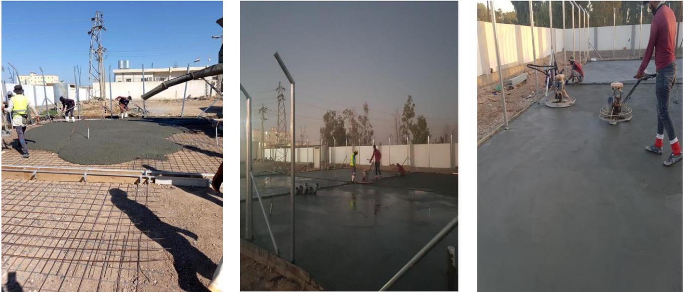
**Workers are pouring concrete slabs for the foundation of the mobile substation.**
